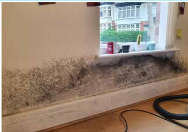
Mould caused by condensation (above)
