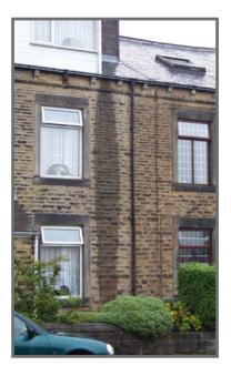
**5.1.2** Rainwater penetration is less frequent in cavity wall construction, but can occur because of inappropriate or poorly installed retrofit cavity wall insulation, mortar drippings, or the cavity being bridged by debris.
