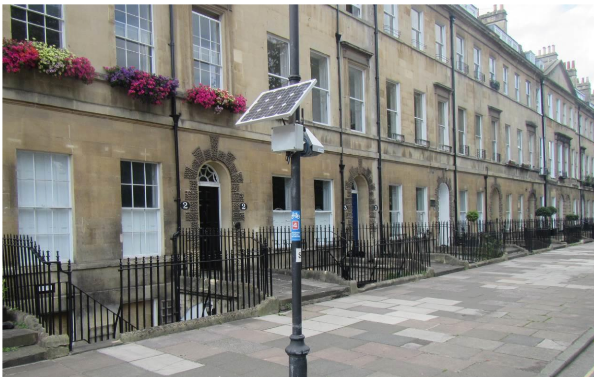
AQMesh Automatic air pollution monitor - Sydney Place, Bath.
