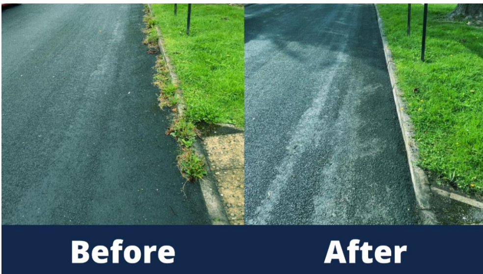
Weeds cleared from pavement on Wick House Close, Saltford ward
