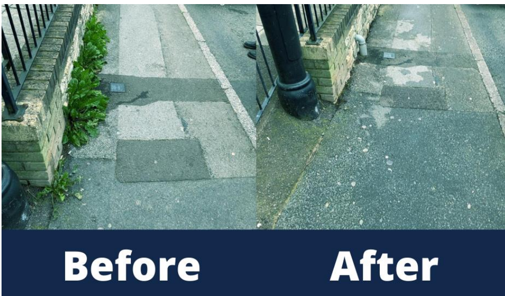
Weed removal completed in Midsomer Norton High Street
