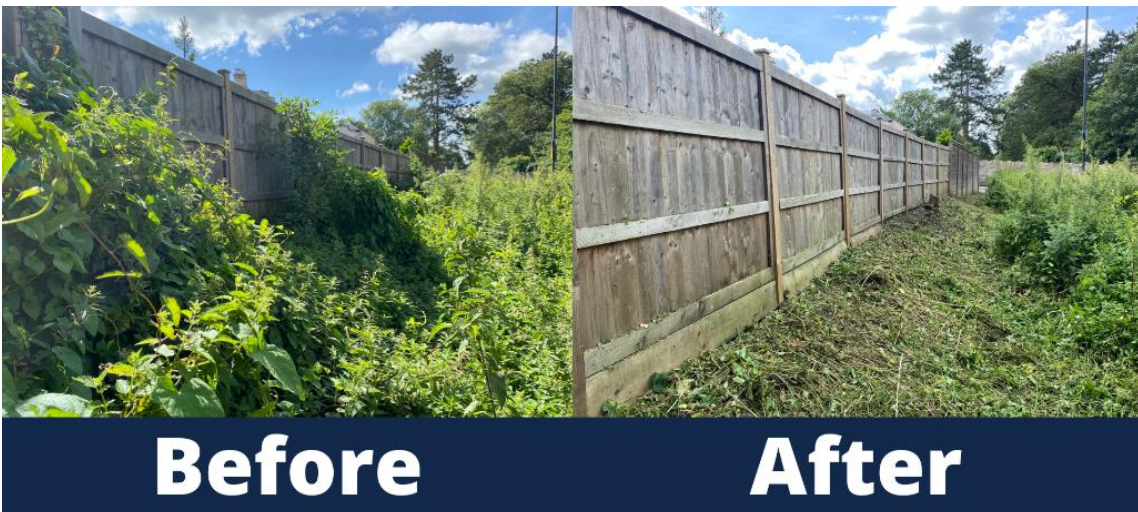
Overgrown vegetation cut away from a fence on Beckford Road, Bathwick ward
