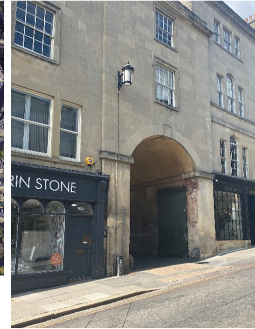
Broad Street Vehicular Access
