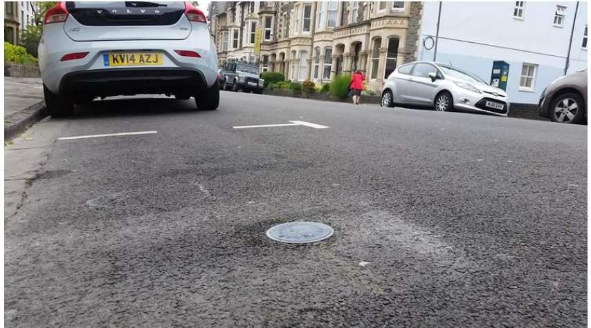
Figure 2-2 - In-Ground Parking Sensors (Source: Smart Parking)
