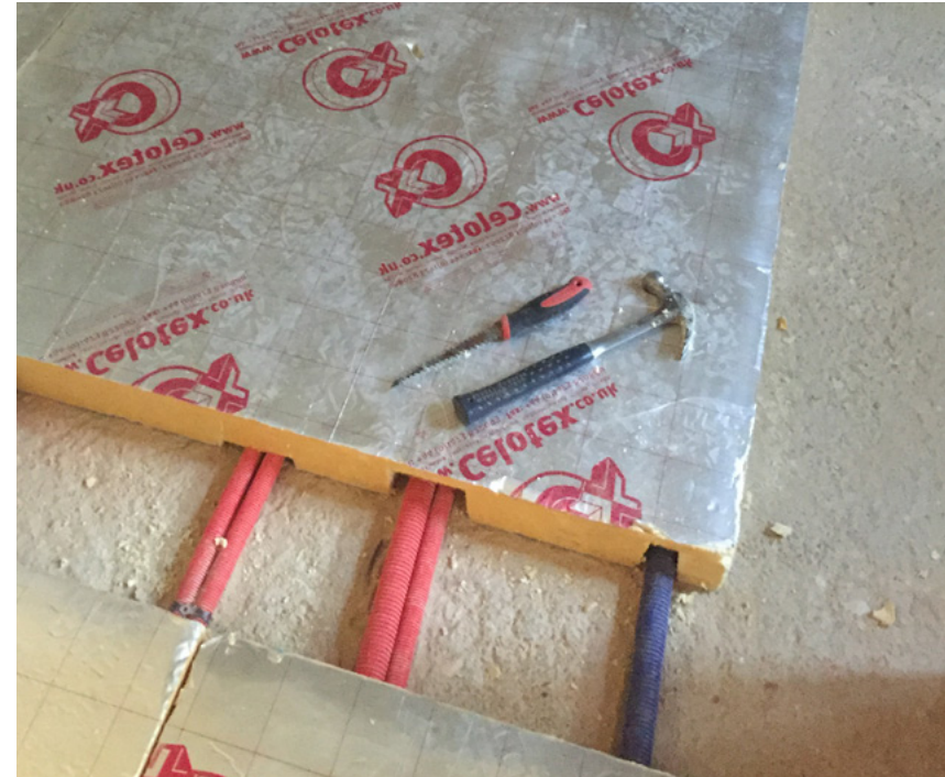
Photo showing insulation with integrated underfloor heating retrofitted to an existing solid floor.
