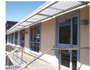
Avoid overheating in summer
