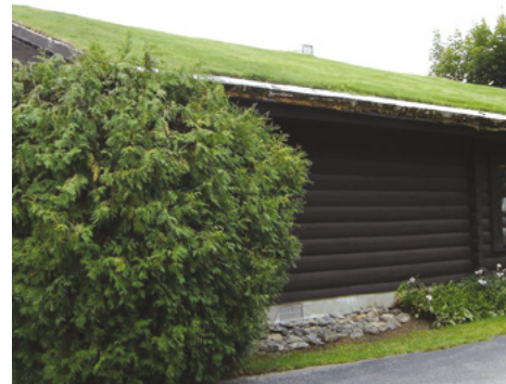
Green roofs can help reduce pollution and surface water run-off and are particularly useful in dense urban areas.
