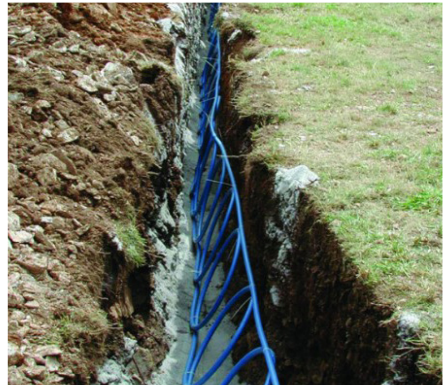
A ground source heat pump slinky awaiting burial. Photo copyright: The Centre for Sustainable Energy.
