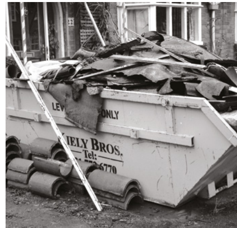
Segregating waste onsite for recycling
