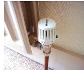
Install heating controls
