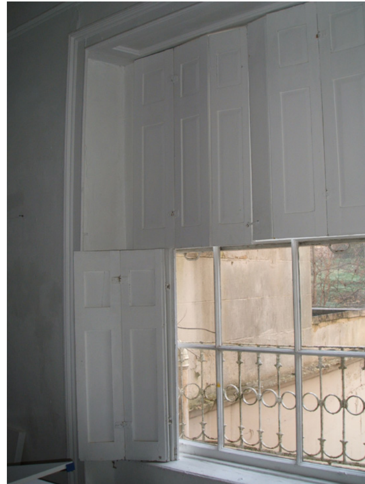
Existing shutters at Somerset Place, Bath
