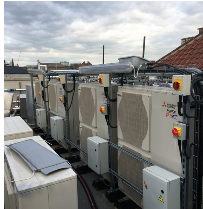
Large-scale air source heat pump installation at roof level.
