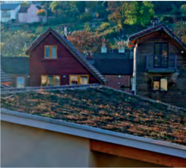
Ashley Vale green roof
