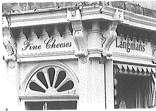
1 John Street (left) Entablature and fanlight over door
