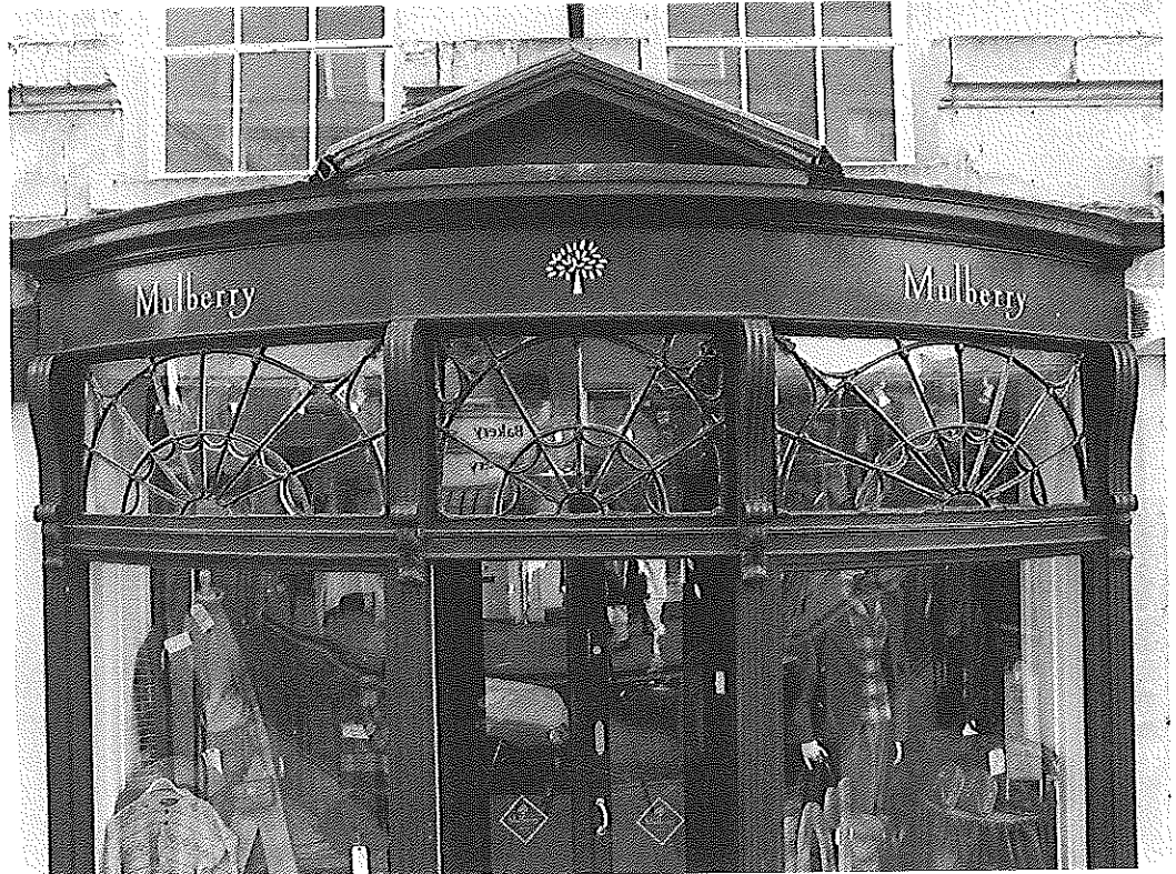
4 Cleveland Terrace [lower right] Quadrant-ended bay showing improved cylinder glass and decorative divisions to upper lights
