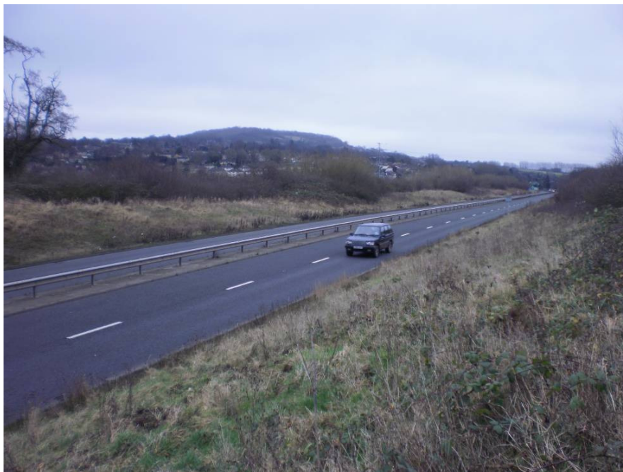
Photo 3.1 View east along the Bathampton bypass at proposed under-bridge location
